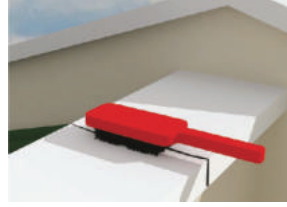
Clean the surface to be used for application
