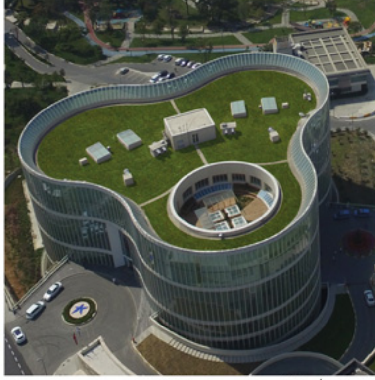
Küçükçekmece Town Hall - İstanbul
