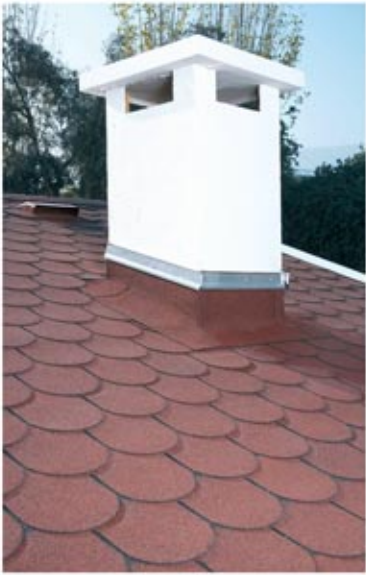
Chimney flashing
