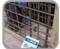
Perde betonunda BTM Swell Bant tape uygulaması / BTM Swell Band application in foundation walls
