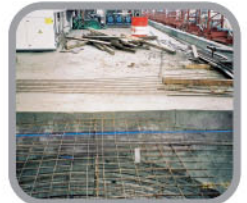
Perde betonunda BTM Swell Bant tape uygulaması / BTM Swell Band application in foundation walls
